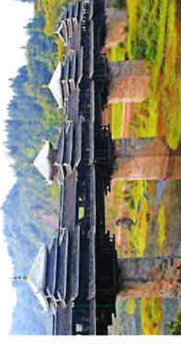
Chenyang Bridge Liuzhou, China
